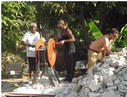
Crushing rubble into usable aggregate
